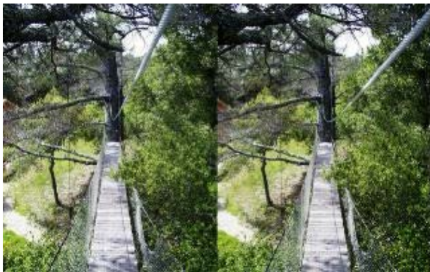
The treehouse bridge from the other side 640 800 1024 1280
